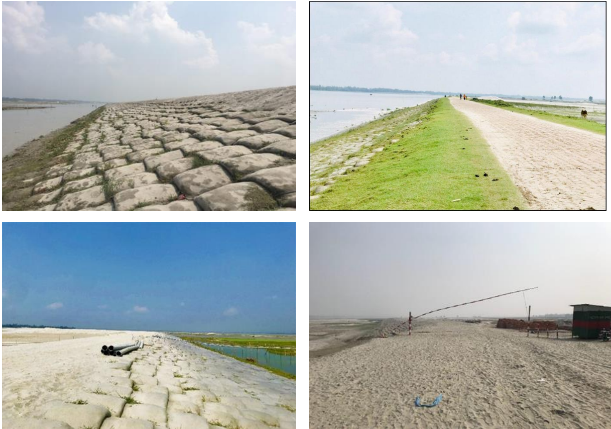
Figure 9: Construction of Embankment.
